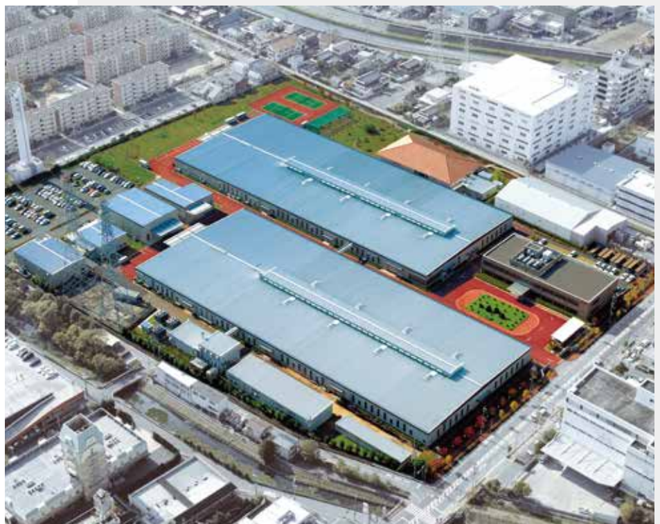
OSAKA-DAITO NEW OFFICE & FACTORY LAND:55,000m 2 BUILDING:27,000m 2
